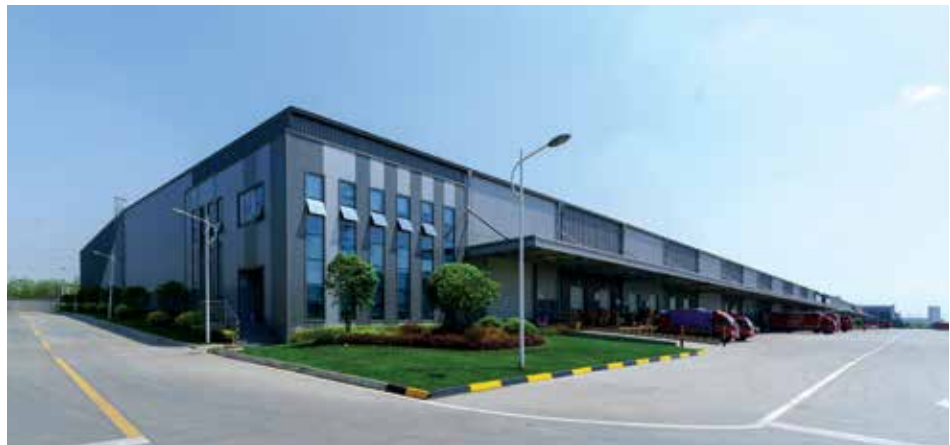
CTF Services issued Green Panda Bonds last year, with the proceeds used for the construction and operational funding of green warehousing projects, including logistics properties located in Chengdu.
